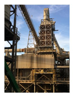
Scheuch Impuls (pulse jet) bag cleaning utilizes low-pressure compressed air, that passes through engineered nozzles and venturis, entraining more ambient air than more traditional pulse jet arrangements. The tuned nozzles ensure that each bag in the row receives the same volume of cleaning air, ensuring even, effective bag cleaning and consistent emissions and pressure drop performance over the life of the bags.
